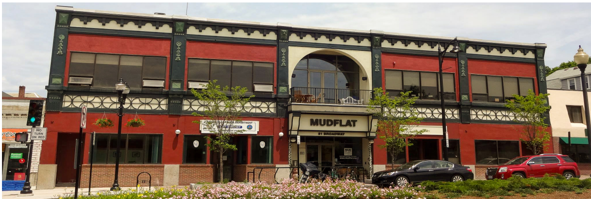
Above: Mudflat Building
